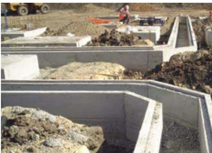
During Construction of Utility Trench
