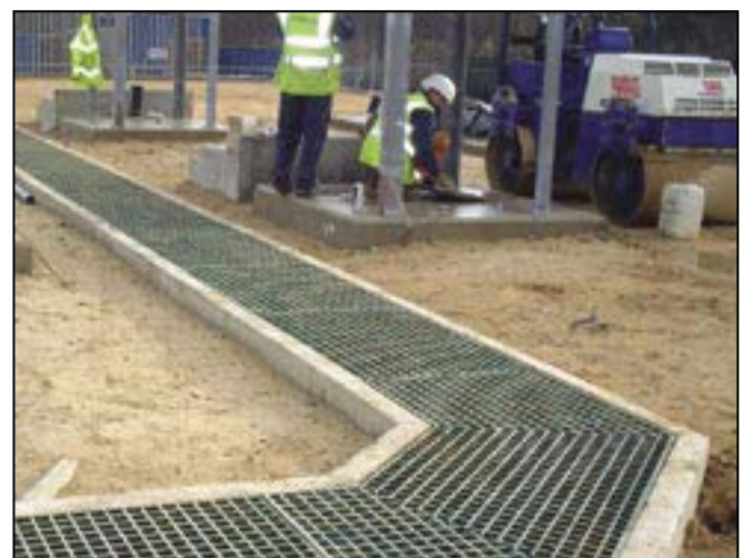
After Installation of FRP Trench Covers
